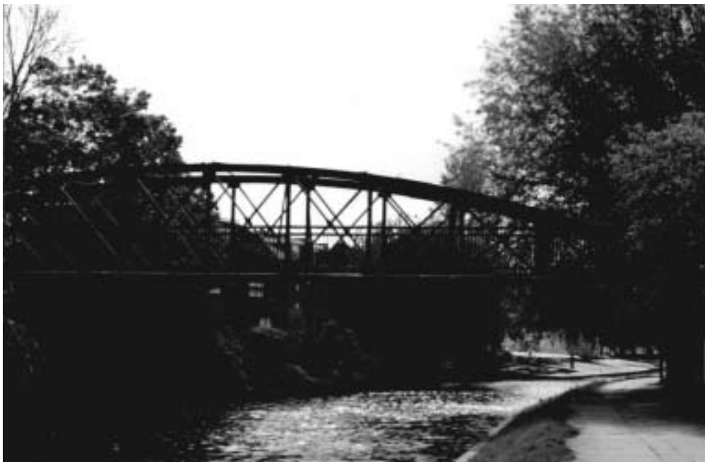
Fort St George Footbridge
